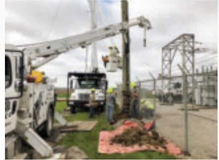
RECC linemen changed out a 70-foot rotten pole at the Lowder Substation. The pole holds the Ameren transmission line “static wire” that is connected to the grounding grid of the substation. It will also serve as a tower/mount for a collector used in our new AMI system.
