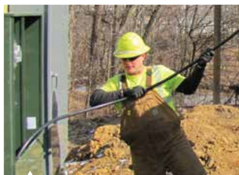
Journeyman Lineman Travis Boylen feeds cable back to the transformer.
