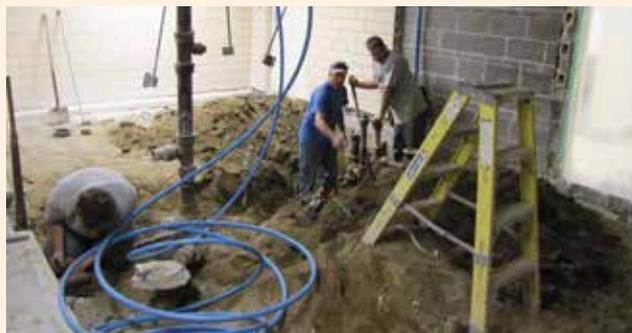
*Workers from Ladage Construction and Snell Plumbing install new piping for the restrooms at Rural Electric's office. New concrete floors were poured in late October. (The space shown will include both the men's and women's restrooms.)*
