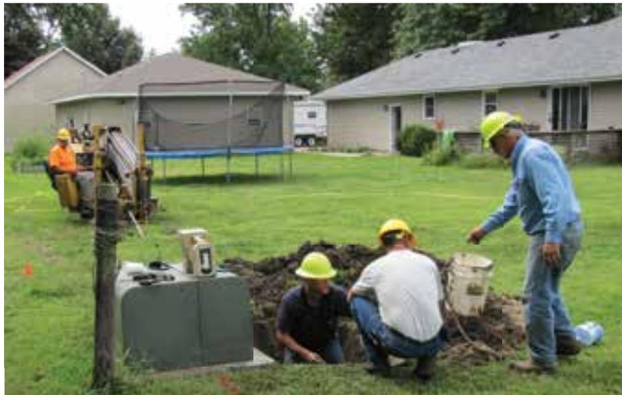
RECC linemen (from left) Travis Boylen, Ken Williamson and Walt Wallace check the conduit pipe being pulled into an excavation by Tom Dickey (background) of ACTS Trenching. They replaced sections of underground cable in the Tower Heights subdivision in Virden using directional boring instead of trenching.
