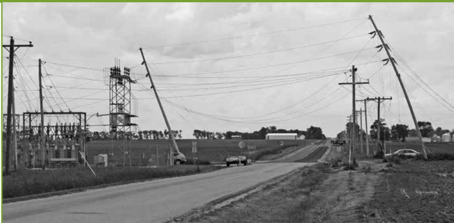
*Ameren's transmission line was knocked down on May 30 along Highway 104, knocking out power to RECC's Lowder and Palmyra substations as well as the towns of Auburn and Waverly. This view is looking south across Hwy 104, along Johns Creek Rd.*
