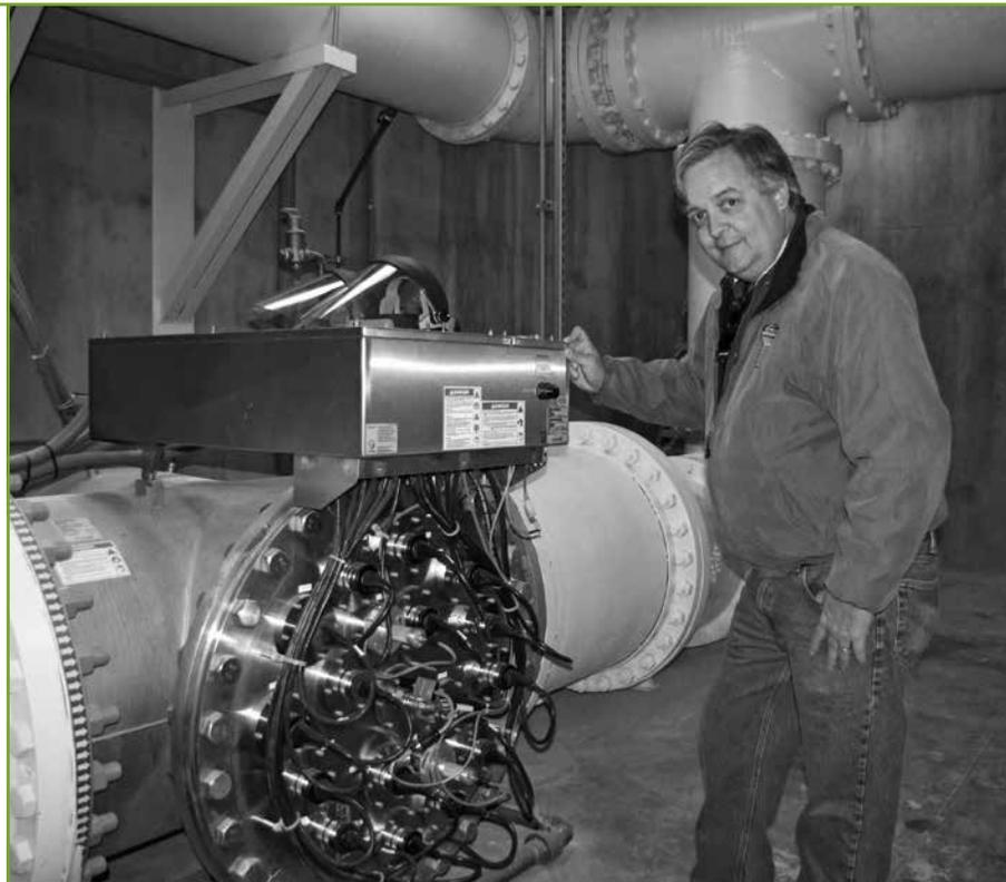
*Dennis Ross, General Manager of Otter Lake Water Commission, checks the bank of ultraviolet lights in one treatment stream at the water plant. The lights are part of a \$2.3 million upgrade project completed at the plant last fall.*
