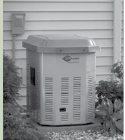
battery if your system has one, and run the generator under load for several minutes to make sure it's operating properly. If you haven't had the engine serviced for a while, have it maintained as needed. Make sure your generator is in a well-ventilated area, and clean any debris that may have accumulated around it.
