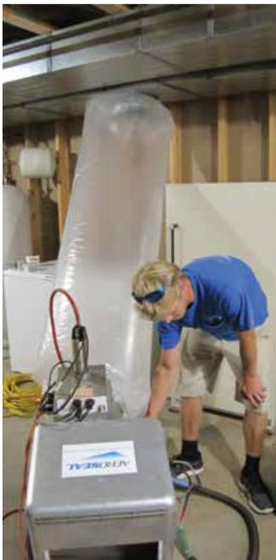
A technician checks the tube connecting the Aeroseal system to the home's main supply air duct.
