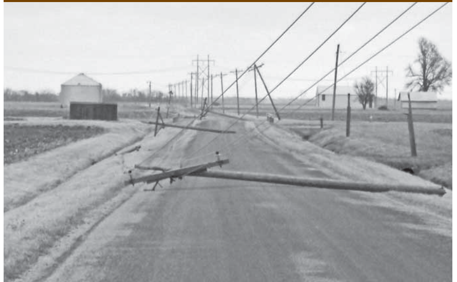
This three-phase line southwest of Kincaid was brought down by high winds on March 8.
