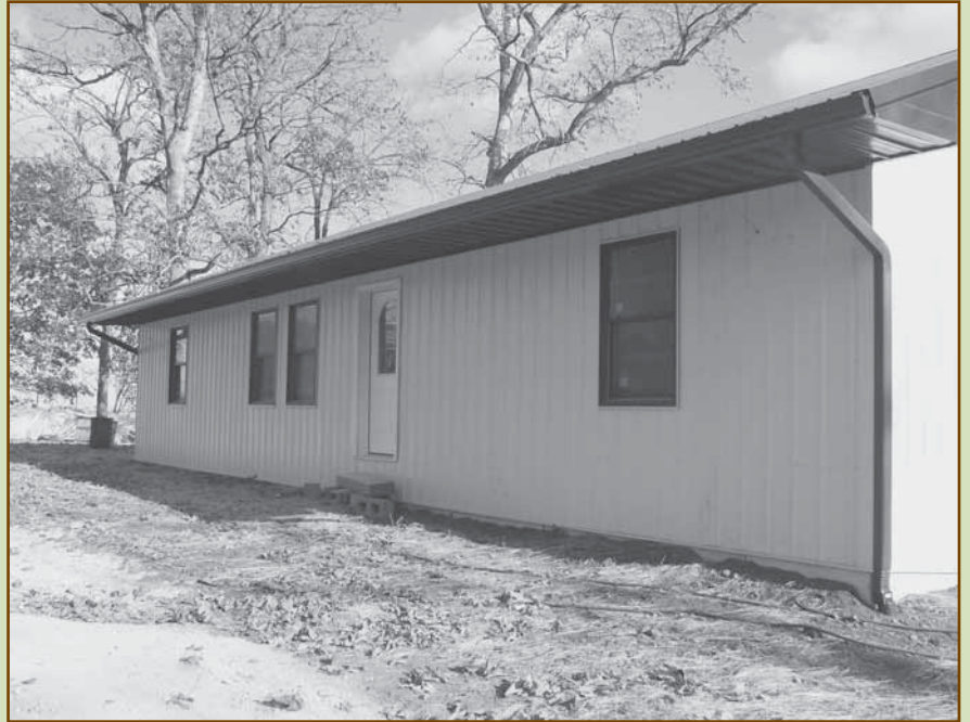
Moe and Jamie Gibbs’ new home east of Palmyra has low-maintenance steel siding and roof panels. Foam insulation and a geothermal heating/cooling system will also help keep the energy bills low.
